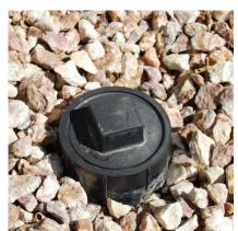
Using a hose, connect а siphon or pump with a capacity less than 15 gallons per minute (gpm) to the access "cap" of sewer cleanout. Run the pump during low-use hours, such as
